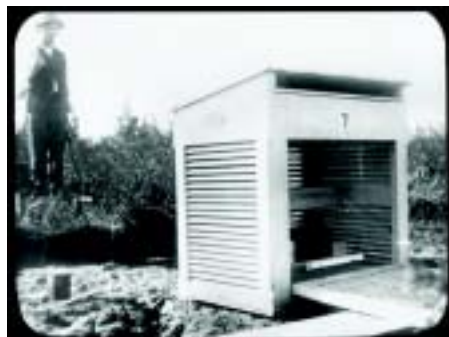
Weather instrument shelter which may have been used in the early days of the Cooperative Observer Program. (Glass lantern slide, circa 1915.)
